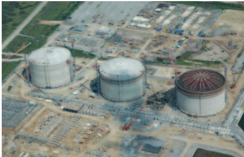
Above: Concrete roofs in place for two storage tanks with the third to be completed in October. Below: The administration building is on schedule for completion in March 2008.
