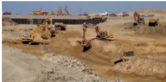
James Construction prepped the site by excavating the clay pit.
